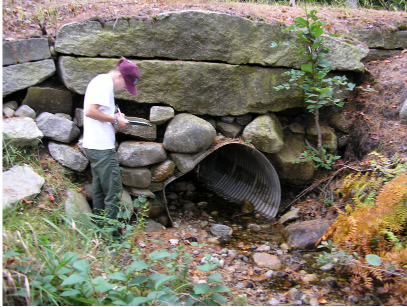
Figure 2. Team member Kirsten Nelson assesses a culvert.
