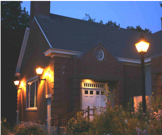
Library facade – fully shielded fixtures provide good illumination where it is needed – on the ground
