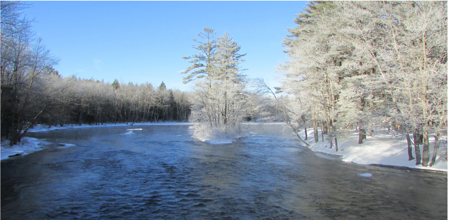
Looking upstream over the Ossipee River on Huntress Bridge in Effingham.
