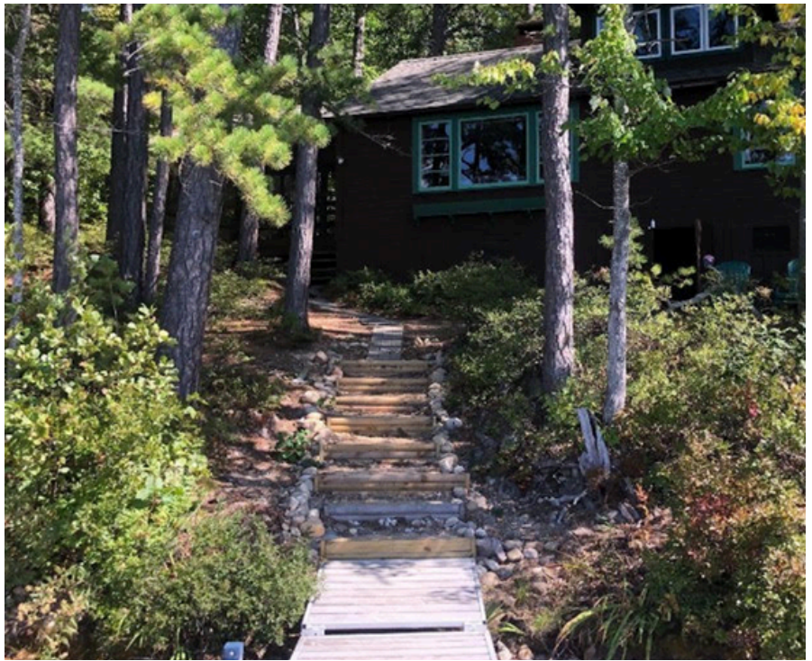
Infiltration steps on a waterbody in the Ossipee Watershed that were put in as part of the LakeSmart program to reduce stormwater runoff and erosion of the shoreline. (Photo courtesy Kat Kelleher, NH LAKES).
